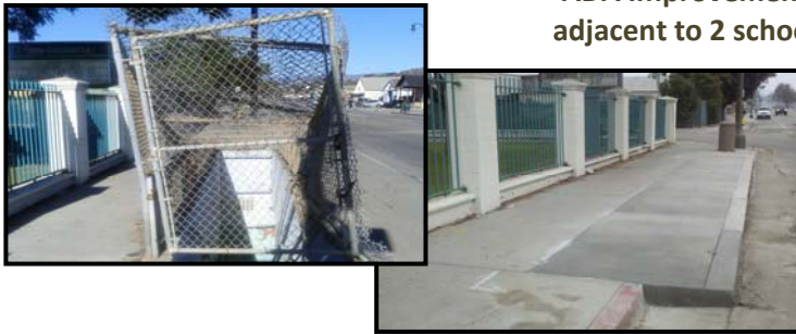
Pedestrian tunnel abandoned & fenced for decades created blighted and unsafe conditions in front of an elementary school. Project included removal of fencing and sealing of tunnel openings, creating safer and more accessible sidewalks.
